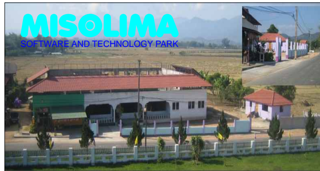
Image shows MSTP under construction
